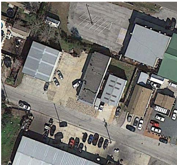
Figure 2. Google Maps aerial view of 33 West 6 th Street. Imagery dated March 2011, accessed online July 22, 2013.
